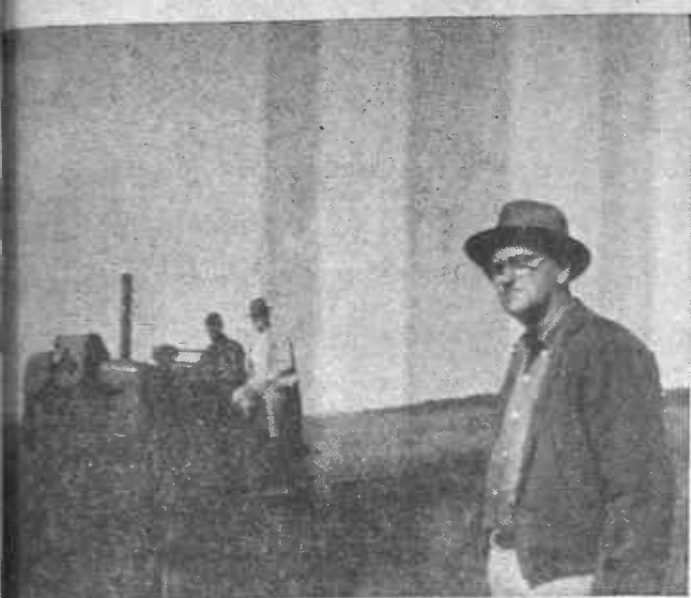
EROSION CONTROL —One method of controlling erosion is vegetating water ways on the Mrs. Flora Bostick farm in the Golden community. Fred Bostick, Sr., right, is shown as he supervised the construction of the vegetated water way that is designed to receive water from terraces and row crops and thus slowing down the flow of water. Operating the bulldozer is Mr. Daily of Red Bay with C. Tice also shown on the machine. This work of soil erosion prevention is carried on through the cooperation of the Soil Conservation Service. Certain financial assistance may be obtained through the county ASC office for practices such as the one shown above. Above picture was made by Hiram A. Jones, Work Unit Conservationist USDA-SCS.
